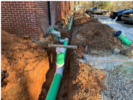
Gutter Drain Tie-In At Gymnasium
